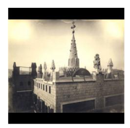
The six chimneys on the upper floor are made of brick, while the 14 on the lower floor are decorated using the *trencadís* technique, using shards of ceramic, glass, marble, vitrified sandstone and earthenware. These elements are a precursor of the *trencadís* pieces Gaudí would create in Güell Park.
